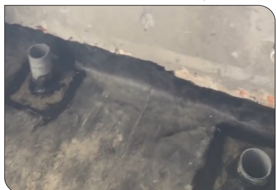
Finish the neck of the pipe and the Baseline corner
